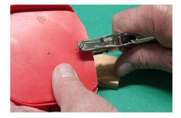
Step 3 (*left*): Thread the retainer onto the machine screw. Done!
